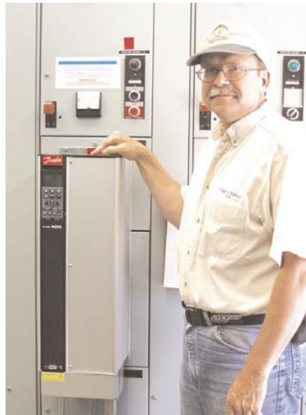
Bob Salmi, Ephraim Wastewater Treatment Facility Plant Manager
